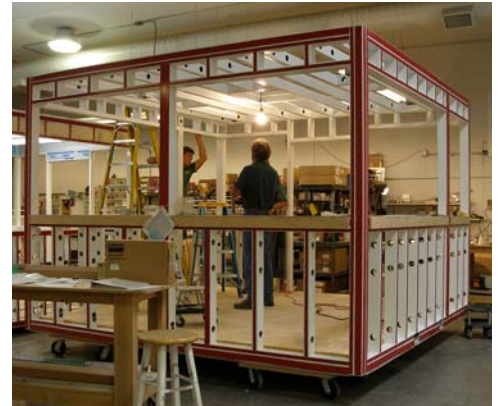
The frame is prepped for electrical
